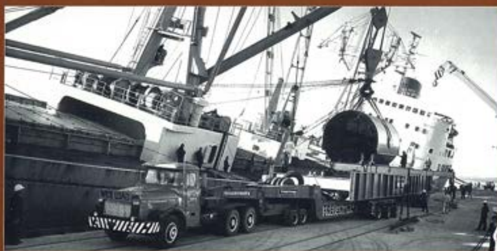
Big George at the New Plymouth Wharf.
